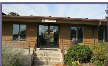
Sycamore Senior Center Golf Course Clubhouse 940 East State Street Sycamore, IL 60178
